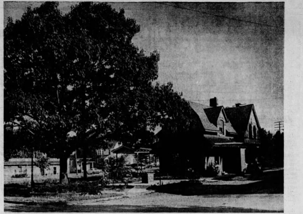
IN PREPARATION for Bicentennial, Wenonah's old train station will become borough hall when volunteers finish renovation.
